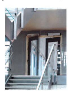
INVERS DFA 127<sup>™</sup> → opens independently with spring tension → safe and reliable also in emergencies cases
