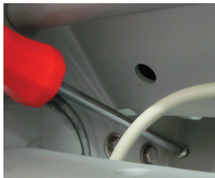
Figure 12: Deck junction box Ejot screws
